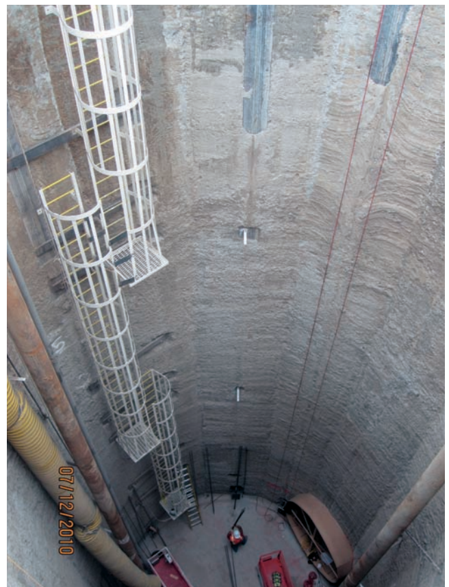
CSM-wall for start shaft microtunneling (USA)
