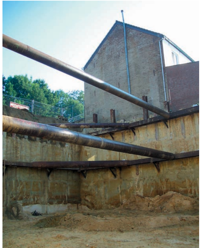
CSM-wall with props (Netherlands)
