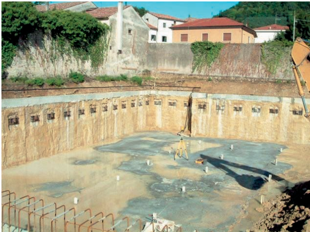
Wall and uplift retention panels with CSM (Italy)
